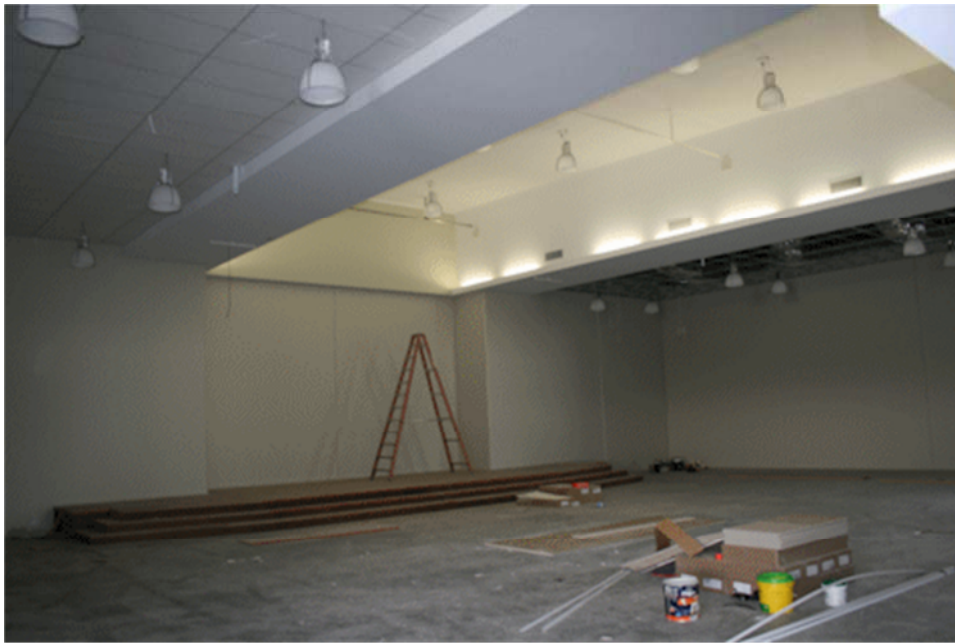
The auditorium now with some of the ceiling tiles in place.
